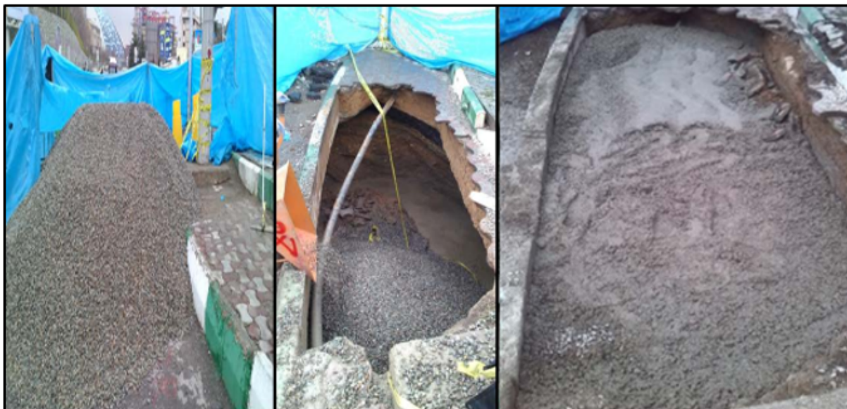
Figure 6. Filled crater by aggregate and concrete.
