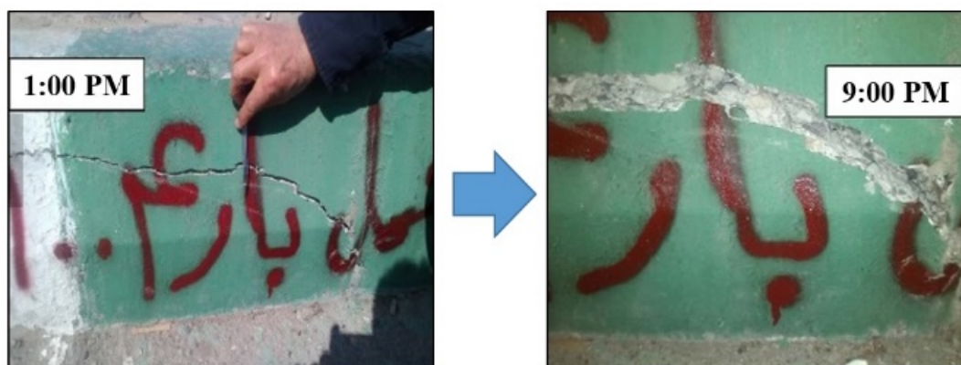
Figure 5. Settlement sign and crack expansion from 1:00 PM to 9:00 PM.
