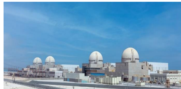
Figure 2. Barakah nuclear energy plant [7].
