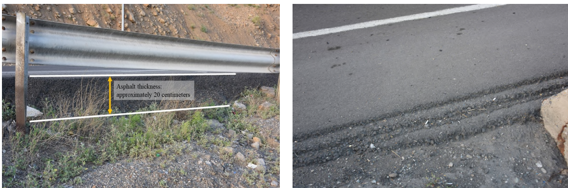
Figure 4. Repaired asphalt in Haraz road passing through the landslide.
