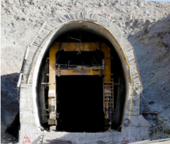
Figure 1. A view of the Miyaneh-Ardabil railway tunnel.
