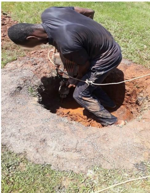
Figure 3. Sinking a well.
